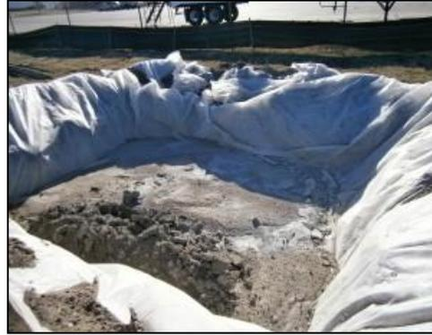
Plate 3-1 Typical concrete wash out areas
